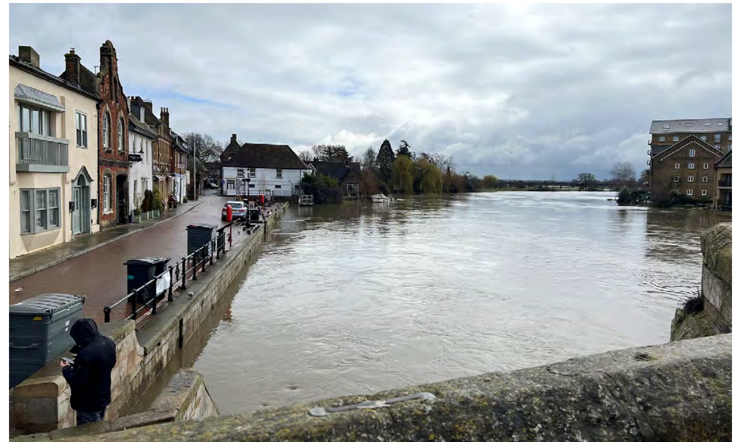
Fig. 16 View east along The Quay
